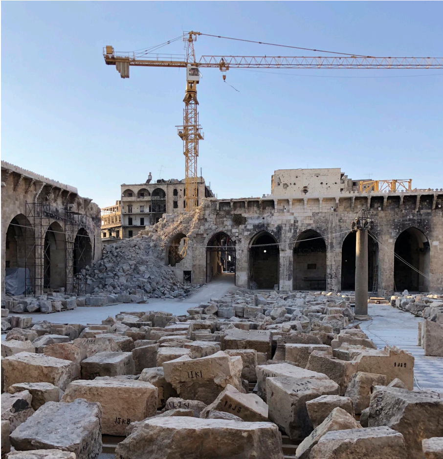
Figure 10.6 Damage to the Great Umayyad Mosque of Aleppo and of the minaret
